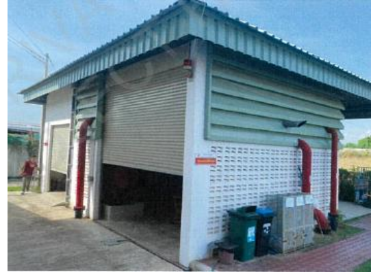
One-storied repair and maintenance building
