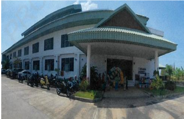
Two-storied office building with garment factory
